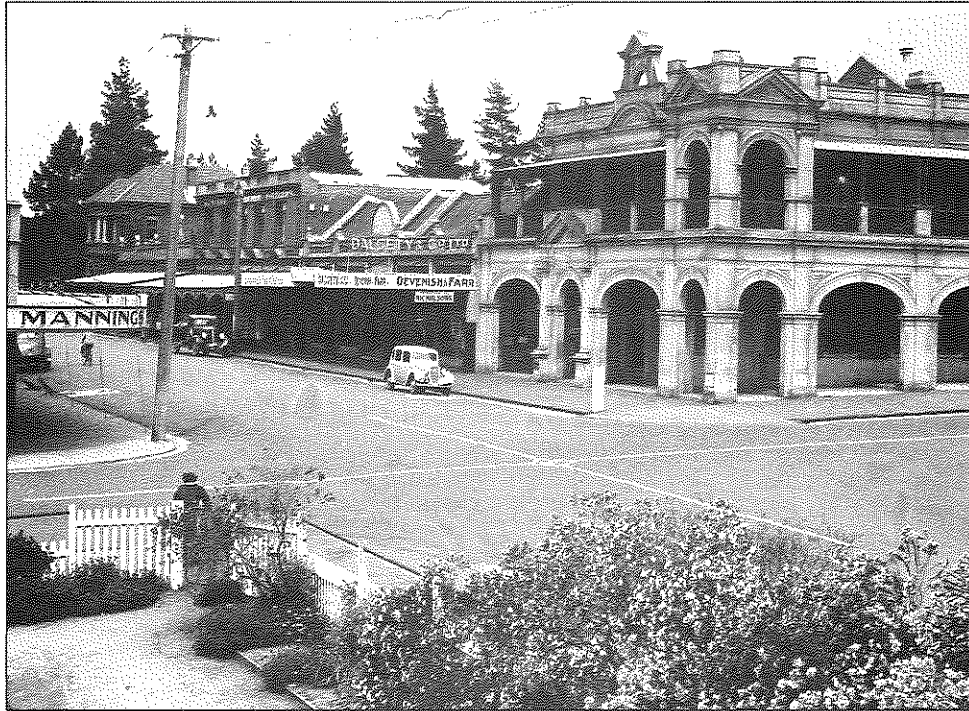
• The Federal Street/Fortune Street intersection (the town centre) in 1930s.
