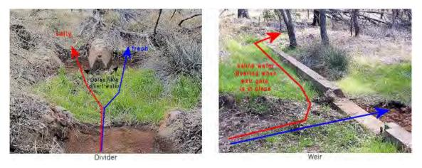
Plate 3: The historical drainage network installed at Railway Dam Reserve (Sawkins 2017)
