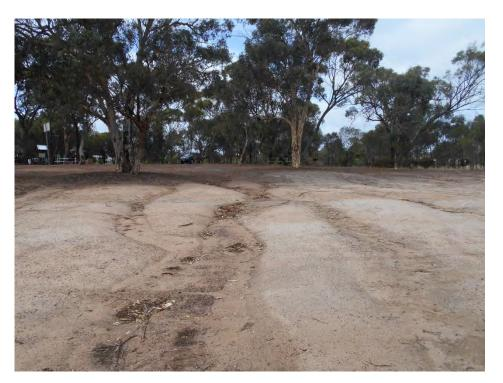
Plate 6: Erosion of banks of Railway Dam
