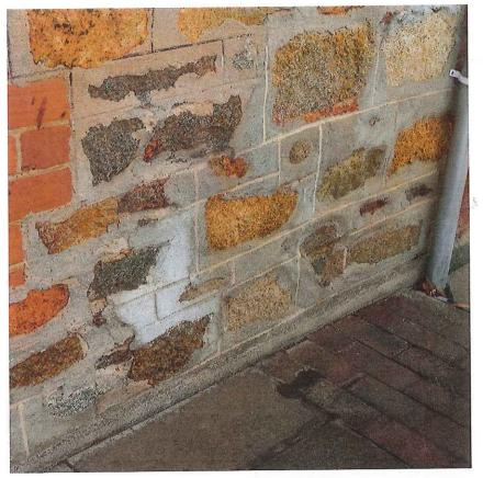
Detail on the south wall showing cement interventions to the face stone near the east corner.
