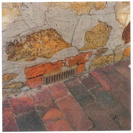
Detail of east wall showing extensive cement interventions and intrusion to air vent at pavement level.
