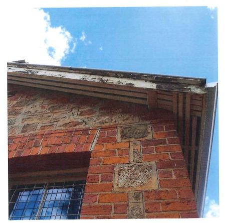
Detail of north corner of east wall showing deteriorated timber and cracking above window.
