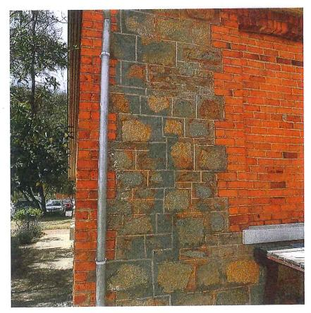
Detail of cement repairs to a full height vertical crack in the west wall at the north front corner.
