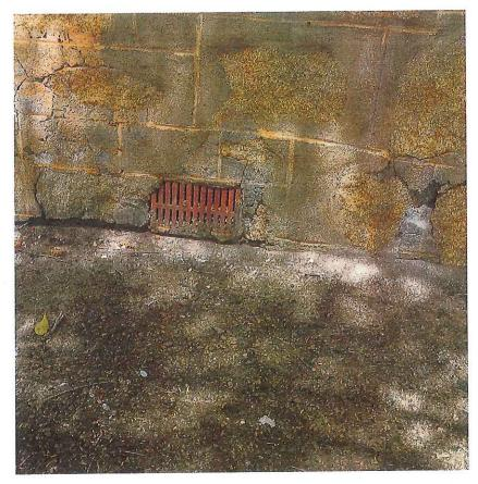
North front wall detail showing cement repairs and raised ground level.
