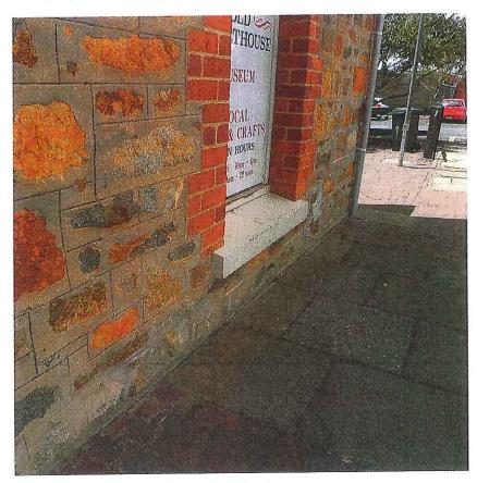
Detail on the south wall showing paving level on the wall.
