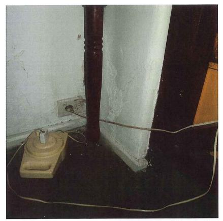
Interior: West wall at juncture of 1895 (right) and 1903 (left) walls showing damp & cracking damage and repairs.
