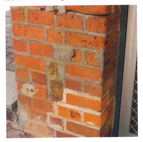
Detail on the south corner of the east wall showing cement mortar interventions to the face brick.
