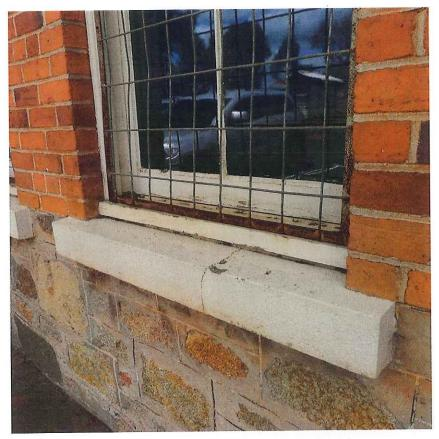
Detail on the south wall showing deteriorated timber window frame, cracked concrete sill and cement interventions to the face stone.
