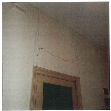
Interior: Room 1 of 1905 addition showing cracks above the boarded door on the north wall.
