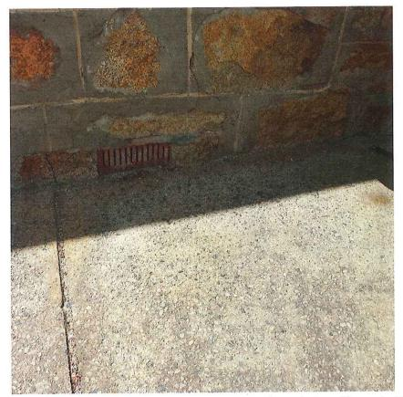
West wall below window 3 showing cement repairs and airvent impacted by ground finish.
