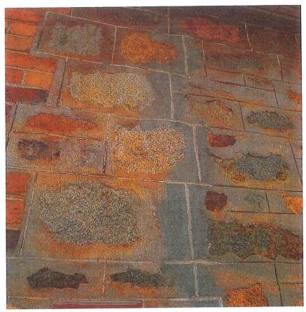
Detail on the south wall showing cement interventions to the face stone the full height of the juncture of the 1903 (left) and 1905 (right) additions.
