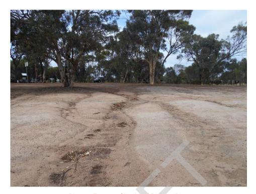
Plate 5: Erosion of banks of Railway Dam
