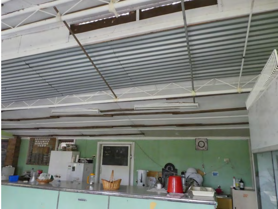
FIGURE 11; TWO LIGHTS IN THE CEILING NEED RE-FIXING MORE SECURELY.
