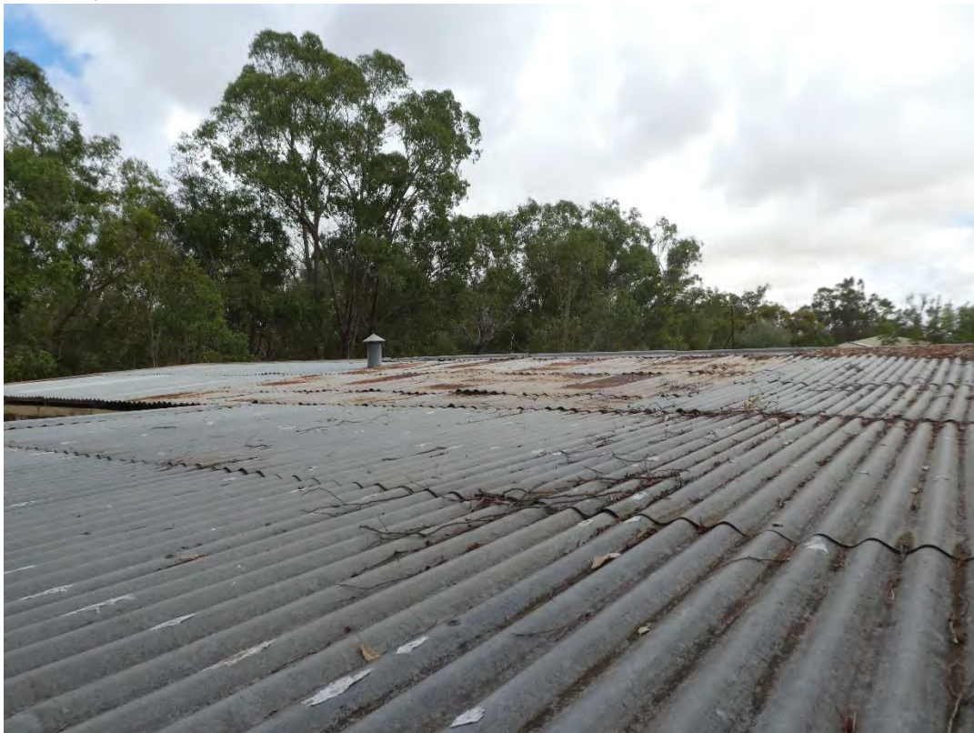
FIGURE 15; ROOF IN POOR CONDITION
