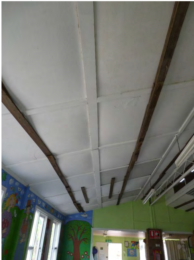
FIGURE 12; CRUDE EFFORT TO ENSURE SAFETY OF CEILING.
