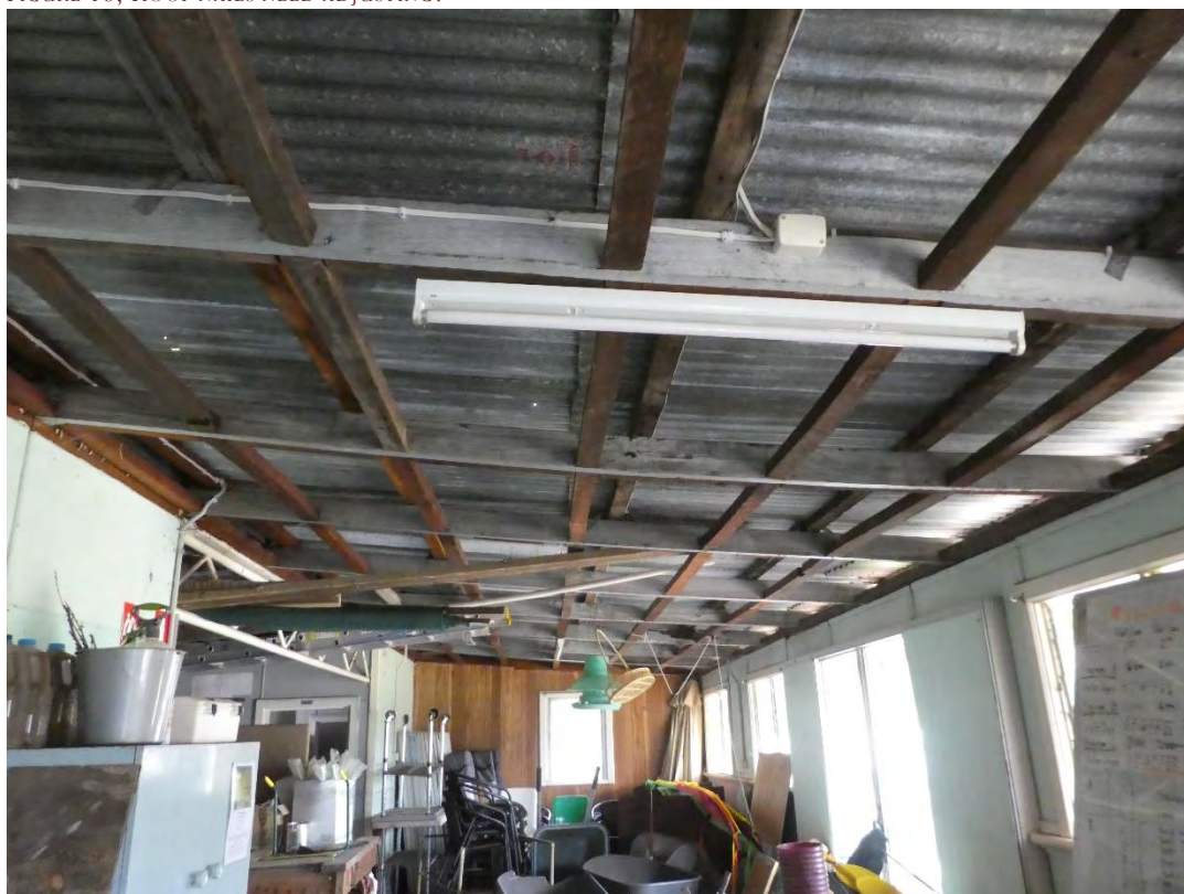
FIGURE 17; SAGGING RAFTERS.
