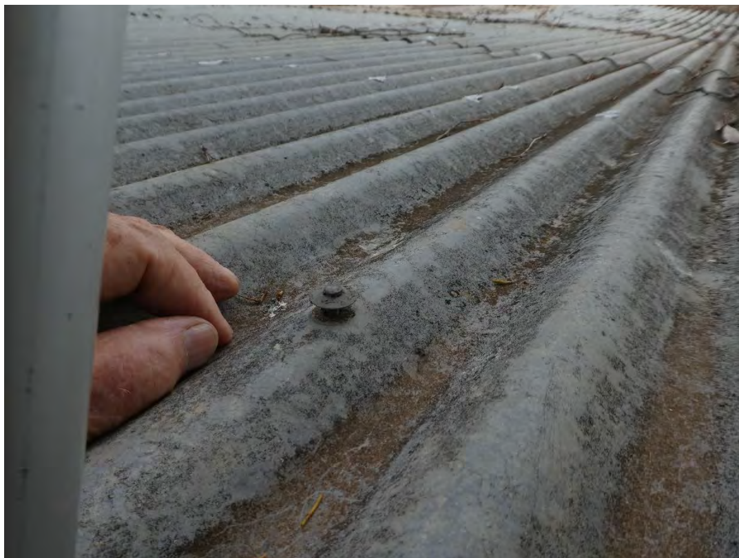
FIGURE 16; ROOF NAILS NEED ADJUSTING.
