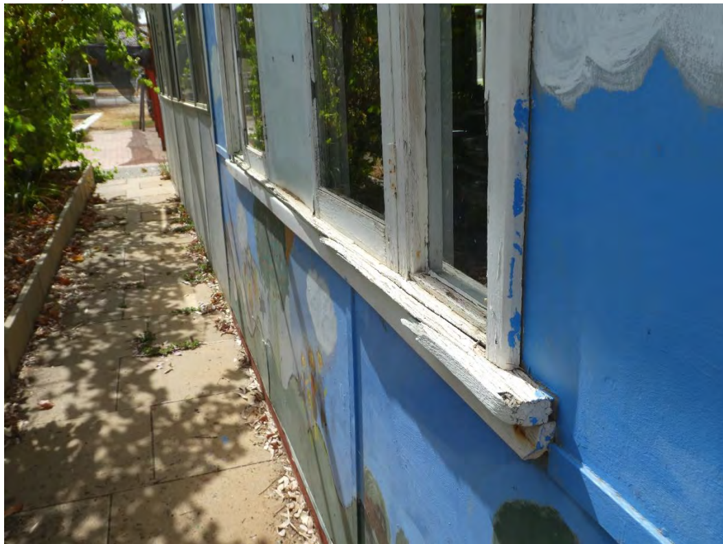
FIGURE 30; SILL COULD BE REPAIRED, IF THE INTENTION IS TO RETAIN AND UPGRADE. THE FAR SILL PROBABLY NEEDS STRENGTHENING.
