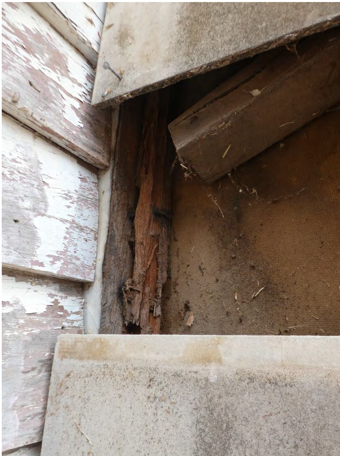
FIGURE 19; TERMITE DAMAGE.
