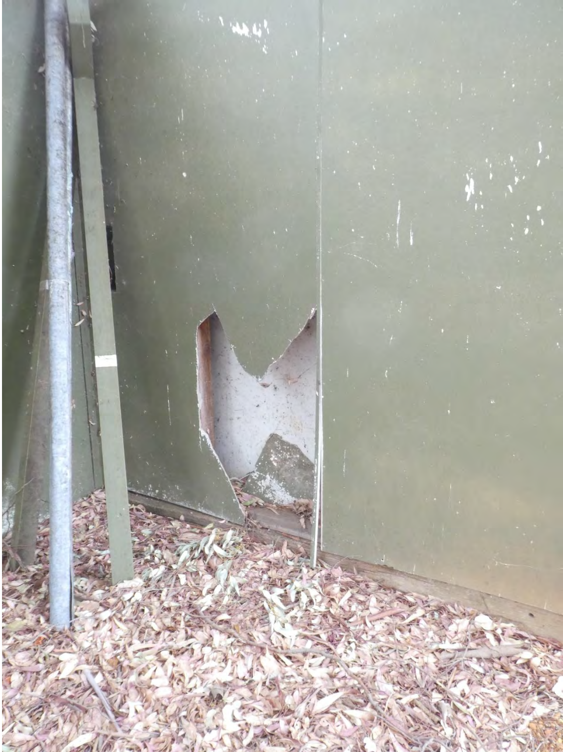
FIGURE 2; DAMAGE TO WALL. THIS MAY BE HARDIE-FLEX.
