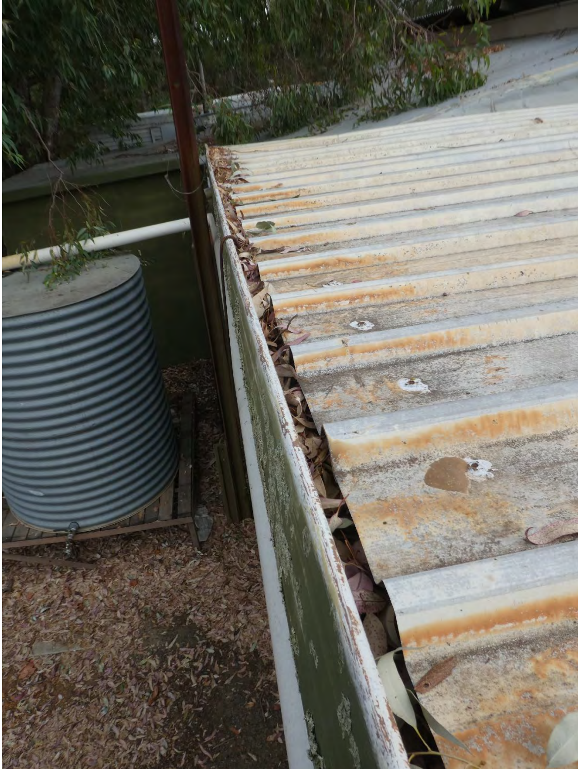
FIGURE 18; GUTTER NEEDS CLEANING. THIS MAY BE CAUSING OVER-FLOW INTO CEILING.
