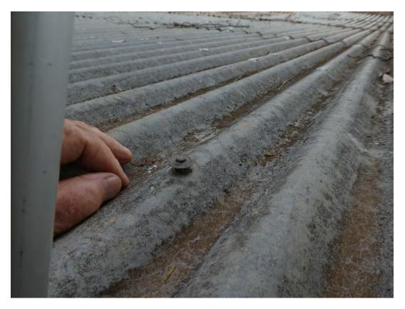
FIGURE 16; ROOF NAILS NEED ADJUSTING.
