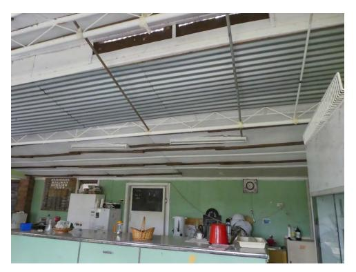
Figure 11; Two lights in the ceiling need re-fixing more securely.
