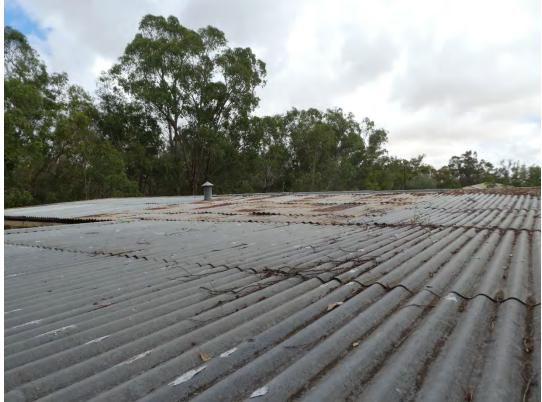
FIGURE 15; ROOF IN POOR CONDITION
