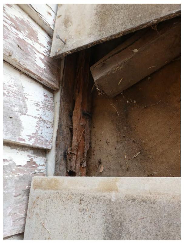
FIGURE 19; TERMITE DAMAGE.
