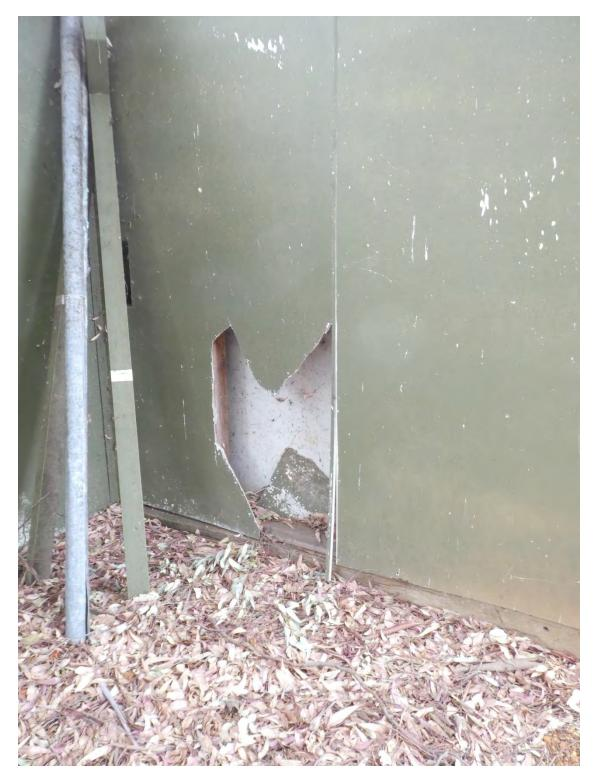
Figure 2; Damage to Wall. This may be Hardie-flex.
